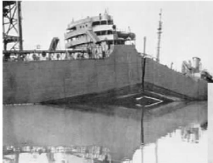
Brittle fracture of SS Schenectady, Jan. 1943
